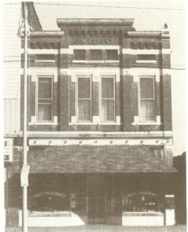
LORENZ BUILDING 2107 West Franklin Street
